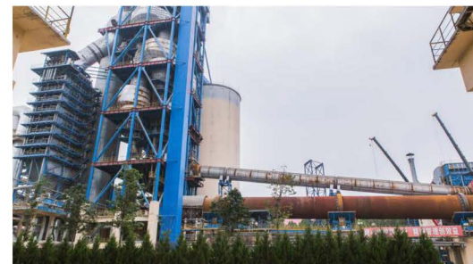
Cement Rotary Kiln
