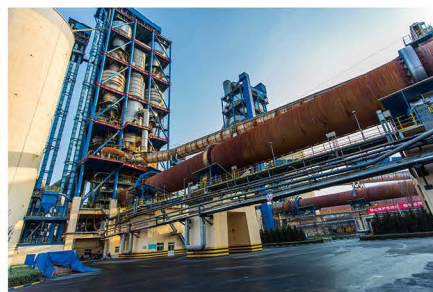
Cement Rotary Kiln
